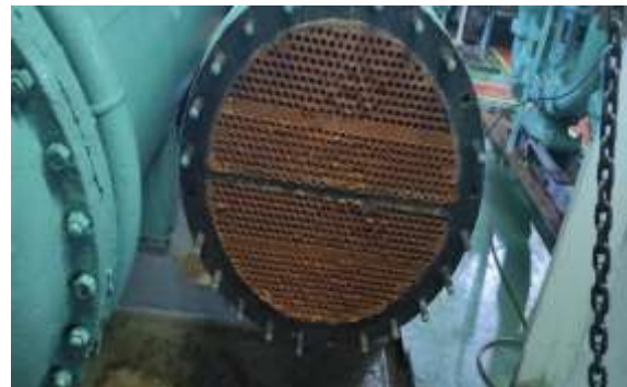
Gambar 4. 5 Pembersihan Fresh Water Cooler
