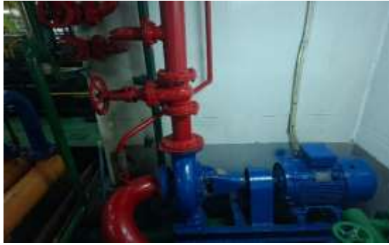
Gambar 8. Fire Pump
